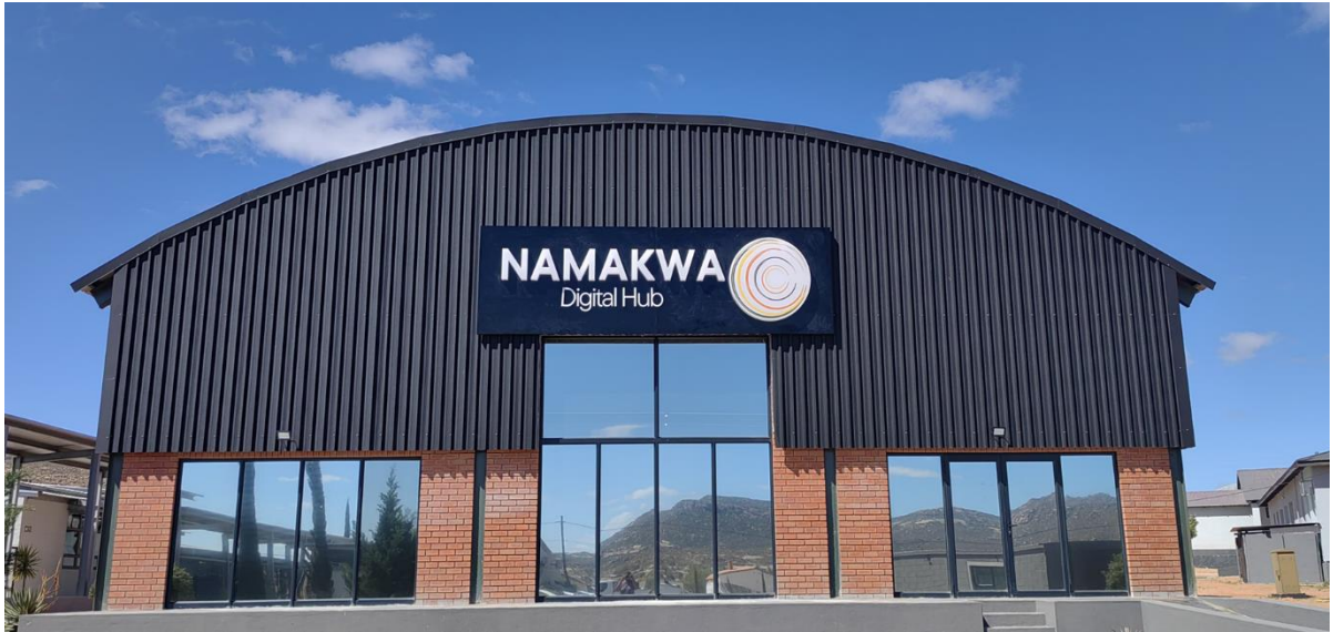
The New Namakwa Digital Hub, Okiep Township
